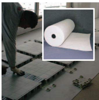
Image 01: Sound Attenuation Blanket (inset) is laid before installation of UniPanels commences.
